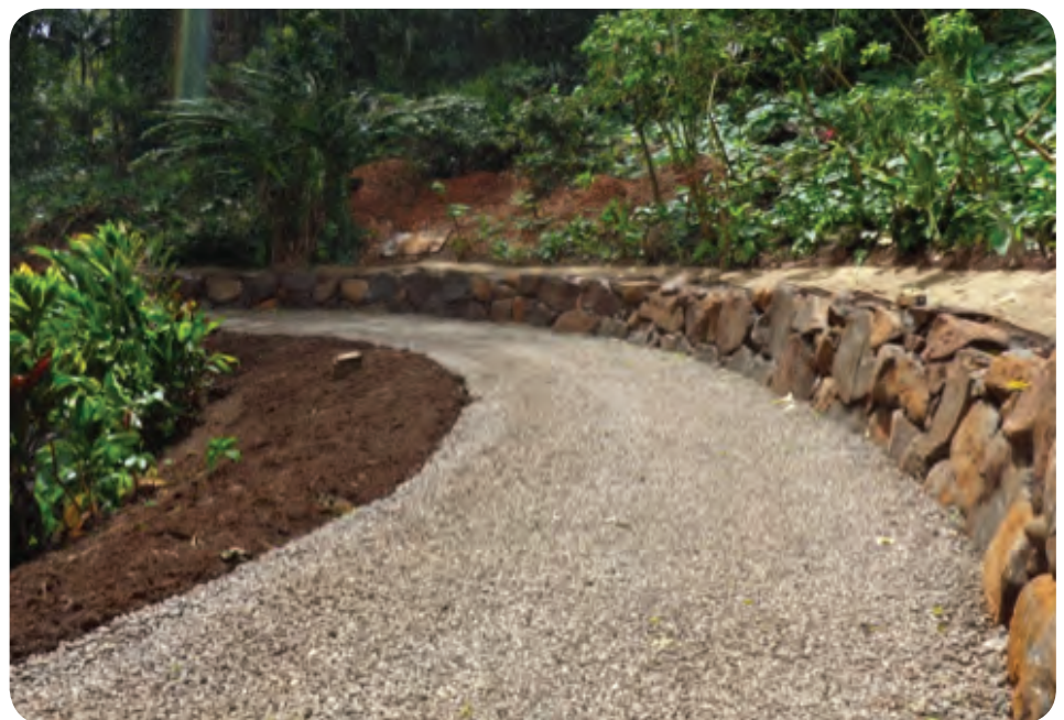
Rock wall and main road at the first big bend.
